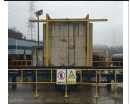
5.N D T inspection
