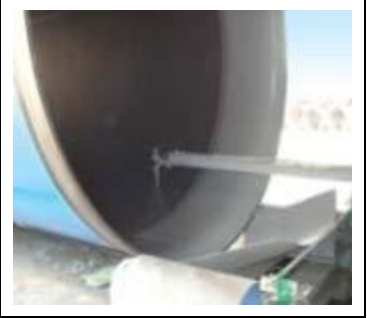
9. Internal coating with epoxy
