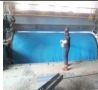
8.External coating with polyethylene
