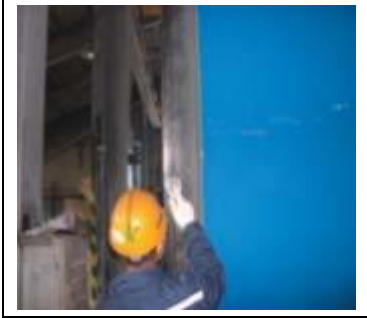
6. Peeling coated film on end part
