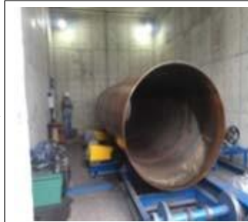
9. N D T inspection
