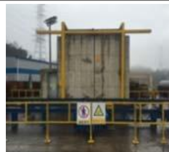
8. N D T inspection
