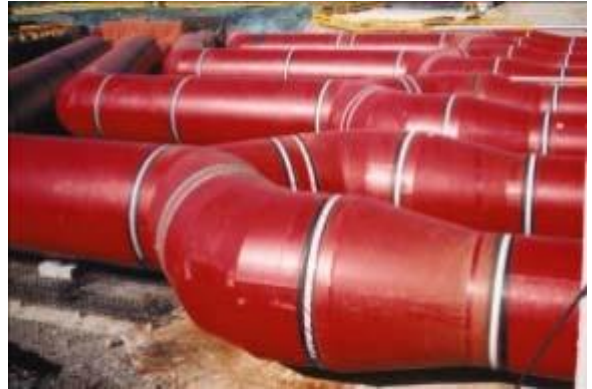
<WATER COOLING PIPE>
