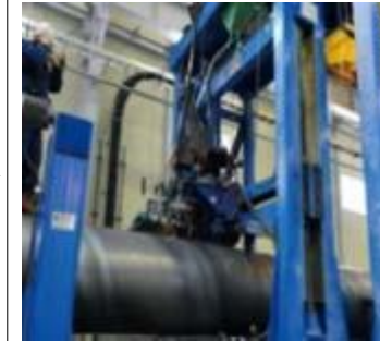
4. Out side welding
