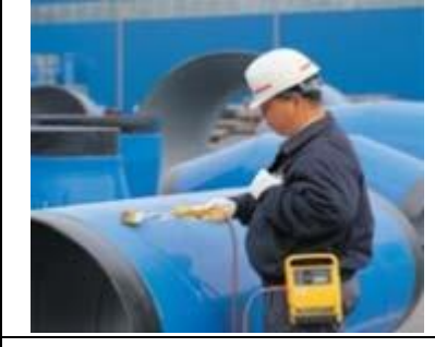
10. External pinhole detection
