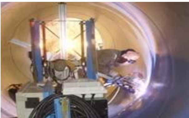
<Automatic Welding system for internal>
