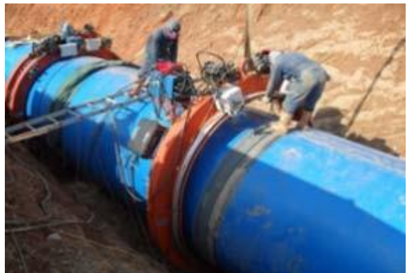
<Automatic Welding system for External>
