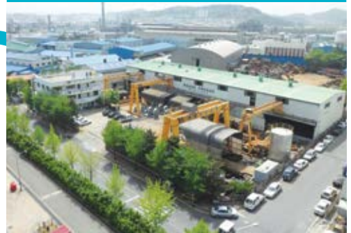
Fabrication Shop No.2
