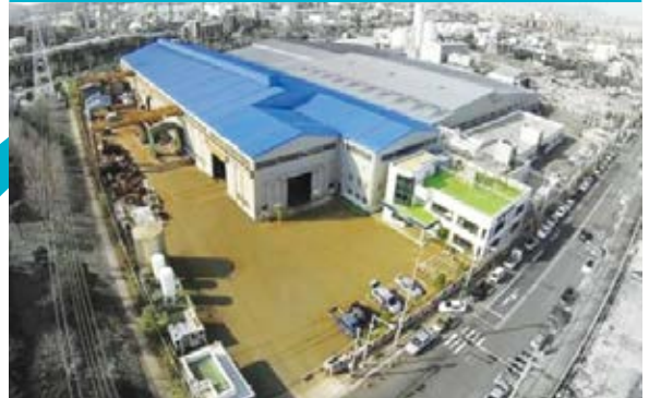
Head Office & Fabrication Shop No.1
